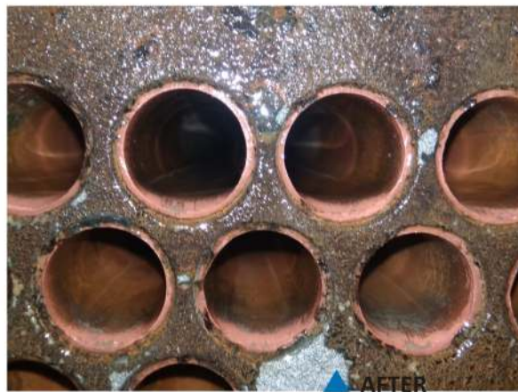
After water draining clean tubes and no scalings
